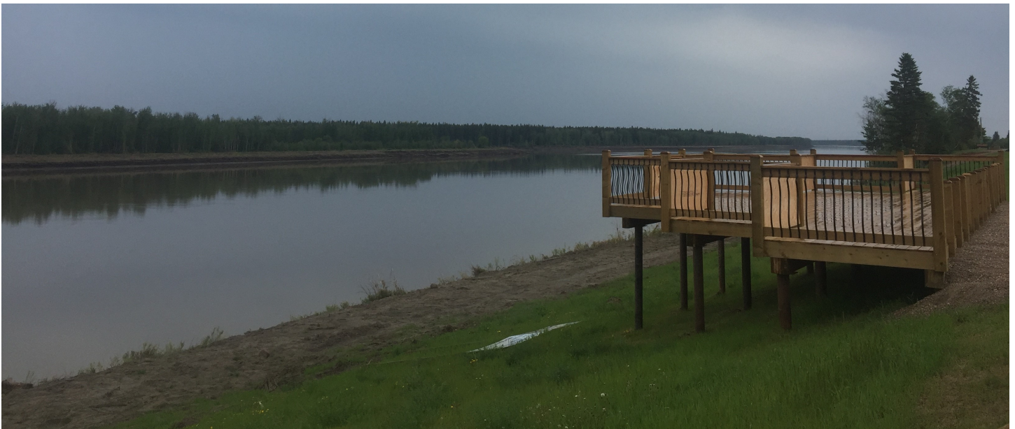
Look-out Deck—Fort Vermilion Streetscape Project
