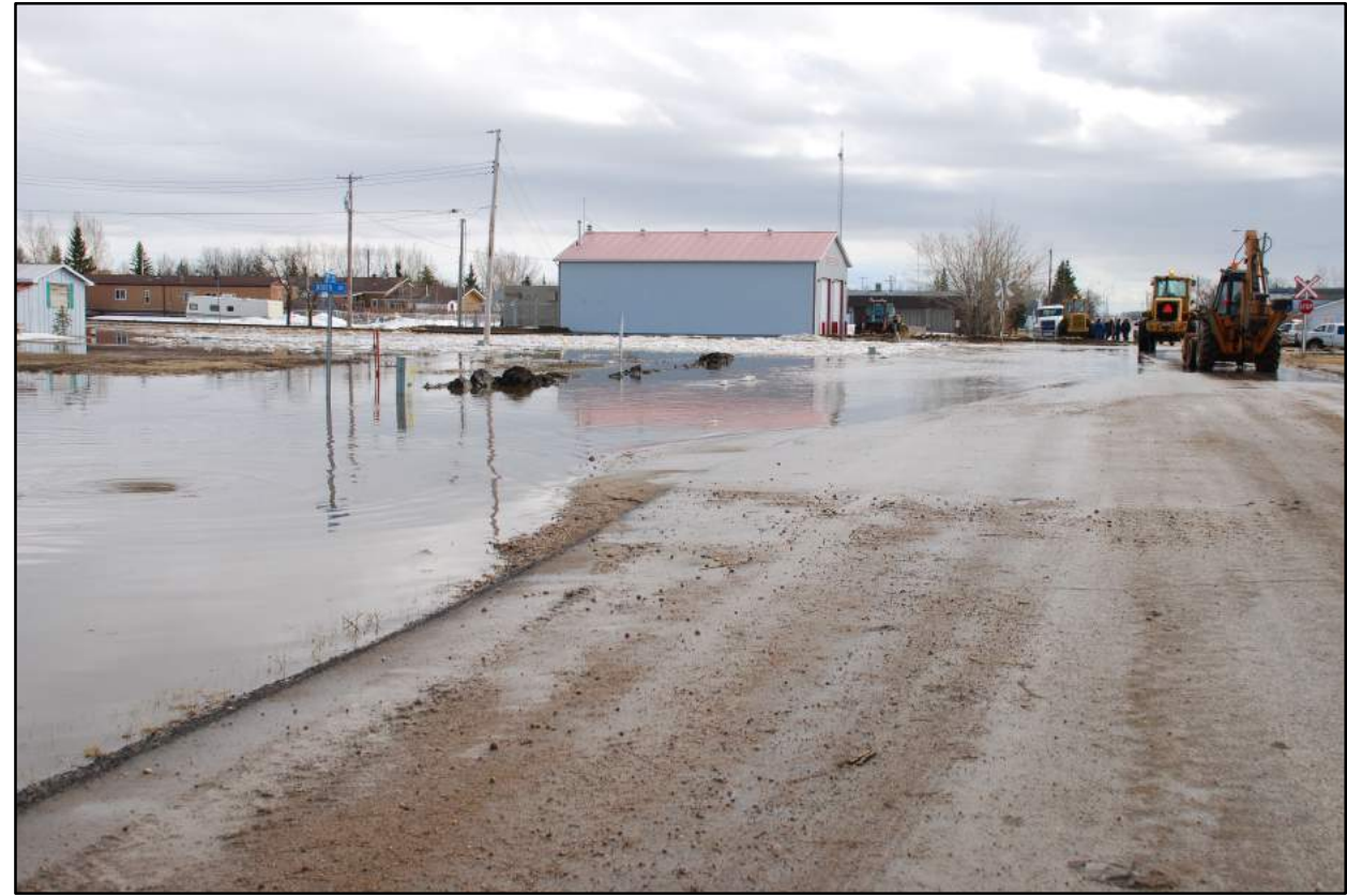
Flooding in Donnelly. Photo taken April 17, 2007.
